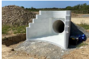
UK's 1st Highways project to use 3D printed concrete
