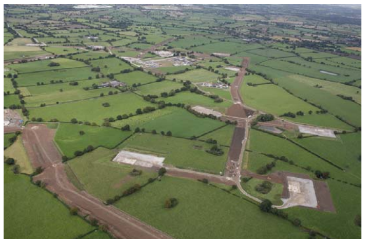
Aerial view of the Stublach Phase 1 Leaching facility showing the well site, infrastructure on a flat Cheshire landscape
