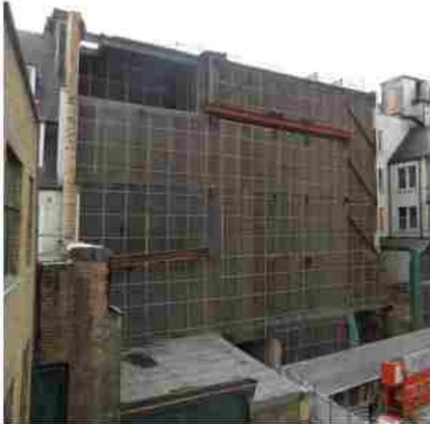
Figure 2.3.3b – Rear of 67-68 New Bond Street
