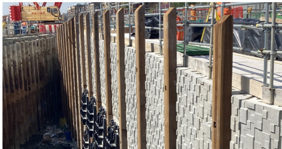
Costain VINCI Construction Grands Projets and Bachy Soletanche JV Thames Tideway East project. The NbS design on the river wall provides a shelving pattern that will allow moisture to be retained, increasing the habitat available for target species within the tidal River Thames.
